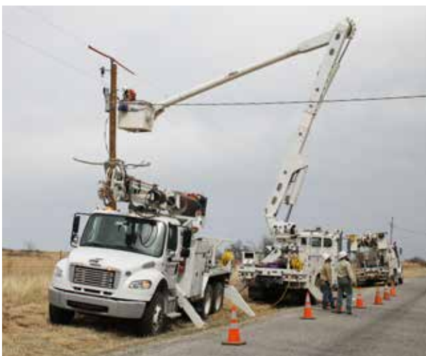
Cotton Electric construction crew sets a new pole near Marlow. Photo by Carli Eubank.
